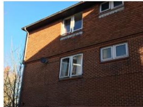
Courtyard materials and treatment.
